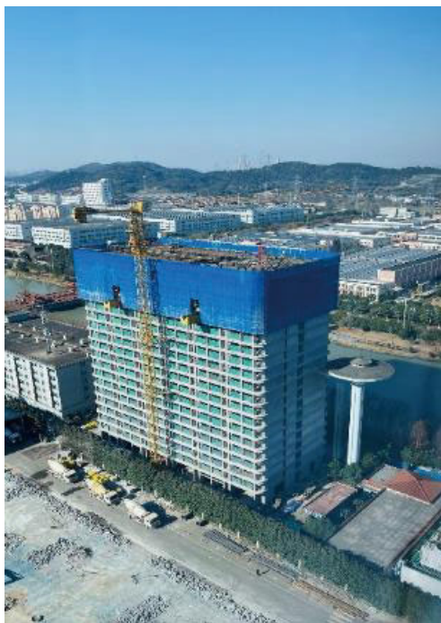
Construction of Haitian Youth Apartment
