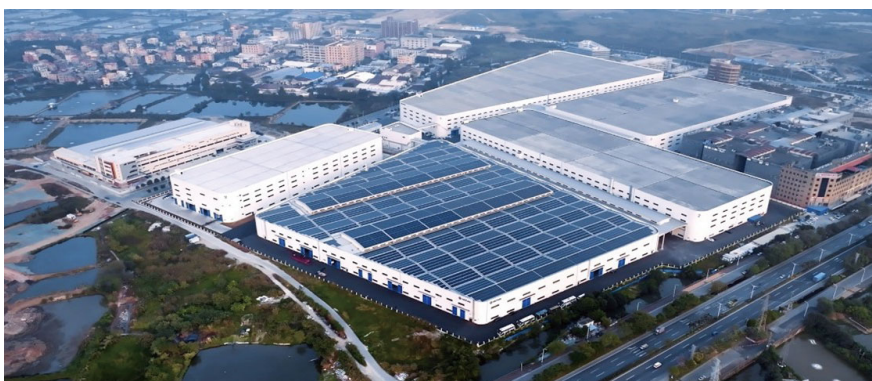
South China Plant PV Project
