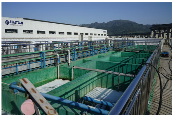
Rooftop Treatment Tank of the Waste Water Treatment Plant
