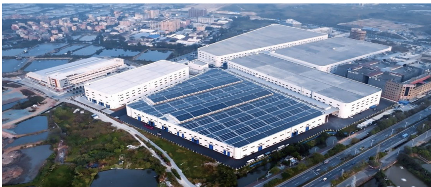
South China Plant PV Project
