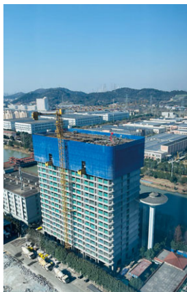
Construction of Haitian Youth Apartment
