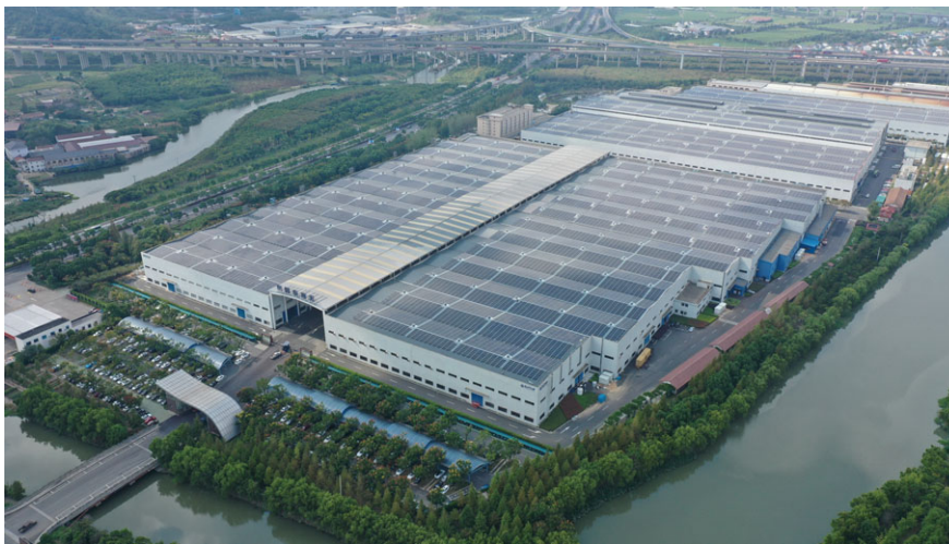
Tongtu Road Plant PV Project
