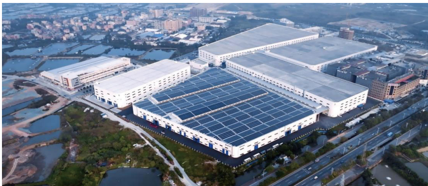
South China Plant PV Project
