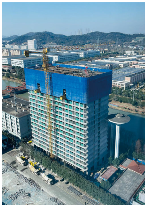
Construction of Haitian Youth Apartment
