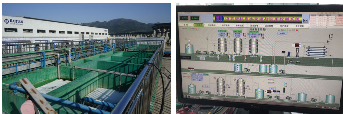
Rooftop treatment tank of the waste water treatment station (left), and waste water treatment and reuse control system (right)
