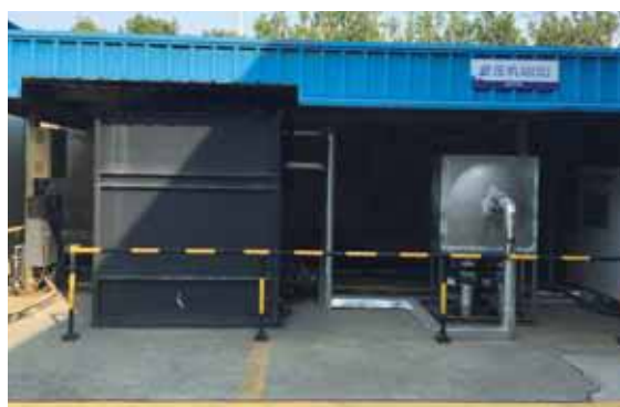
Recycling system of cooling water
