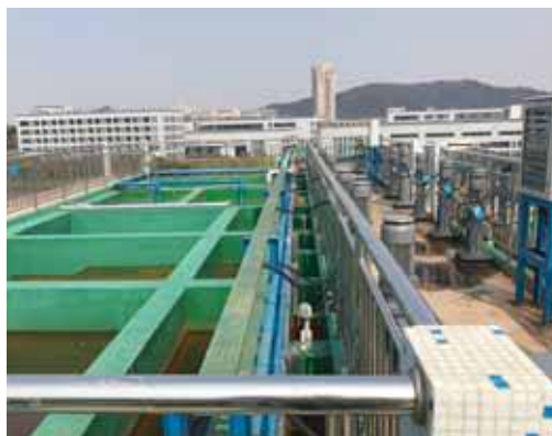
The sewage treatment plant in one of our factories in Ningbo, China
